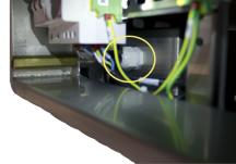
The cable gland is located near the bottom of the cabinet.
