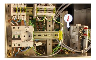
For these models you have to remove the fibre optic splice box to remove the power module.
