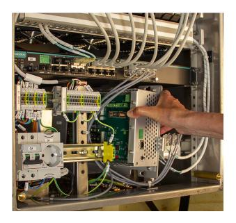
8 Older models of the x82 transceiver will not get past the fibre optic splice box.
